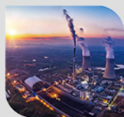
Environmentally friendly heating
