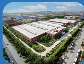
Laishan Industrial Park
